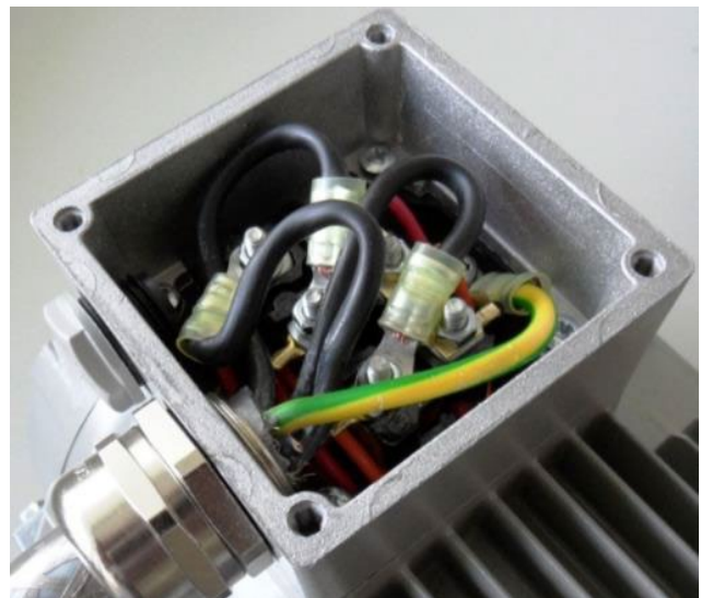
Fig. 32: Wiring on the motor connection box
