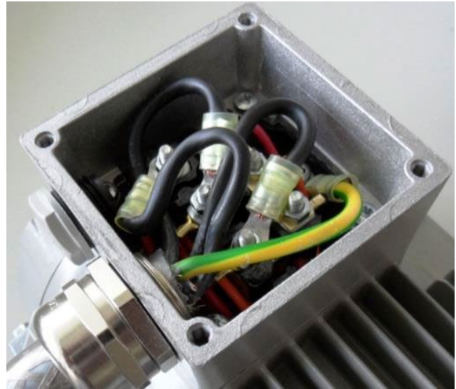
Fig. 25: Wiring on the motor connection box
